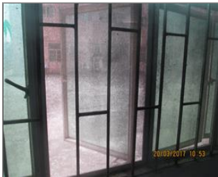
Photo of the canteen (if applicable) The mosquito screen had been installed for the kitchen area.JPG
